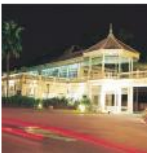
Historical Building & Structural Lighting
